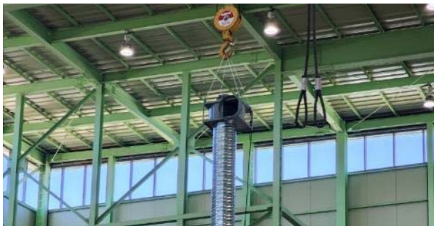
Figure 3: Installation of ventilation fan
