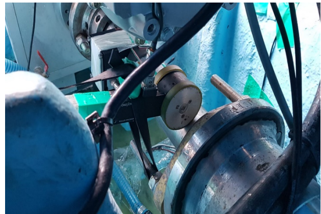
Figure 6: Roller encoder installation at propeller shaft for angular velocity measurement
