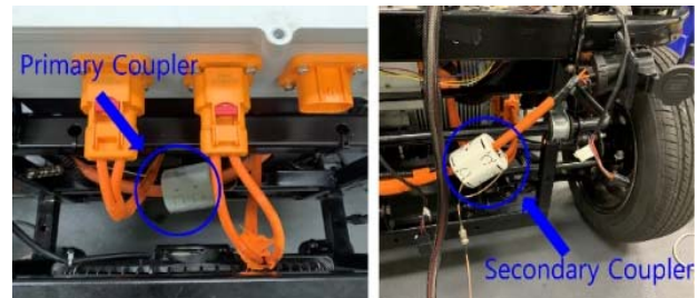
Figure 4: High voltage battery – External charger experiment configuration
