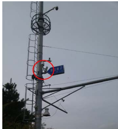
Figure 3: A roadside station used for WAVE communication
