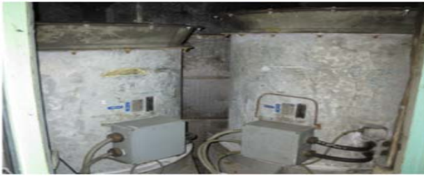
Figure 3: Engine room fan of MT Suula
