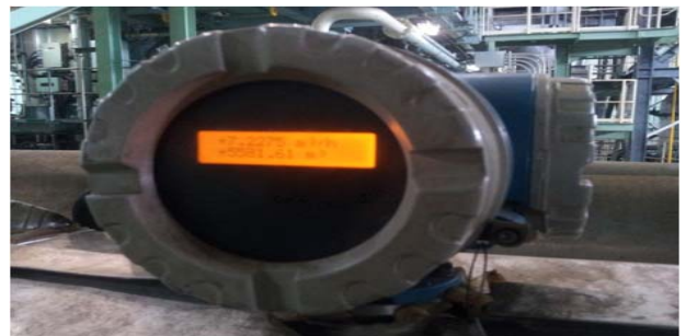
Figure 7: Fuel flow meter
