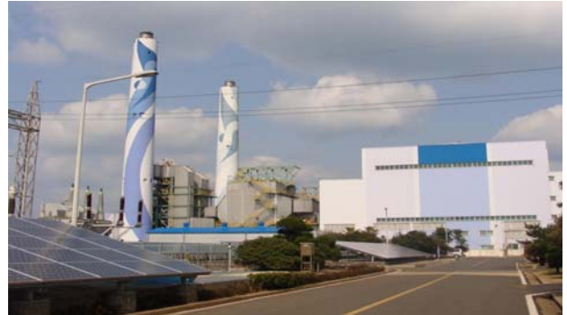
Figure 1: Thermal power plant
