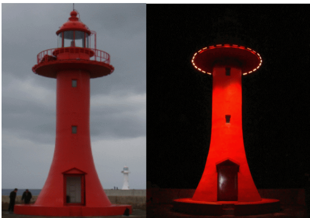
Figure 11: Pictures of breakwater lighthouse installing LED floodlight (Seogwipoehang in Jeju Island).
