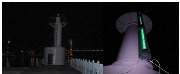
Figure 9: Photograph of the original lantern and installing LED Light Pipe (Green)
