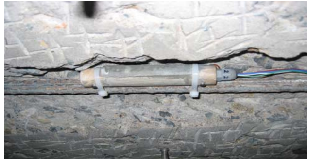
(b) Installation of sensor
