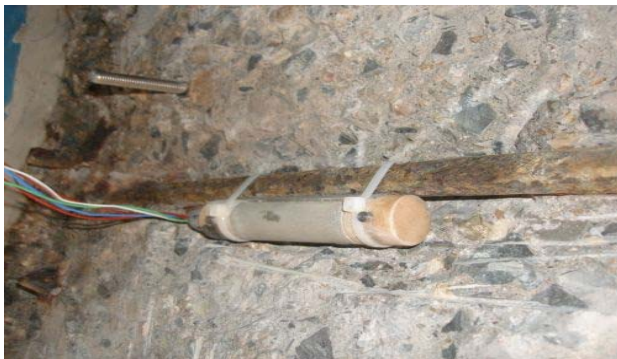
(b) Installation of sensor
