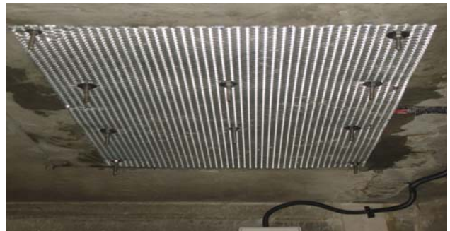
(c) Installation of anode
