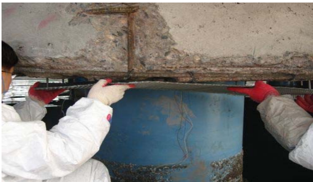
(c) Installation of anode
