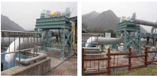
(b) Installation image-A (c) Installation image-B
