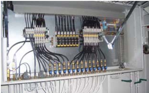
Figure 1: Central system for hydraulic controller
