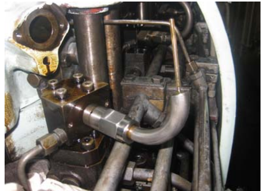
Photo 1: Injection timing measuring tool using high pressure pipe
