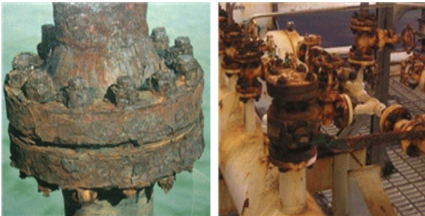
Figure 2: Galvanic Corrosion
