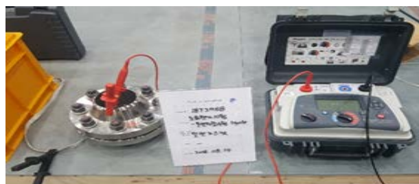
Figure 9: Insulation resistance test and polarization index test
