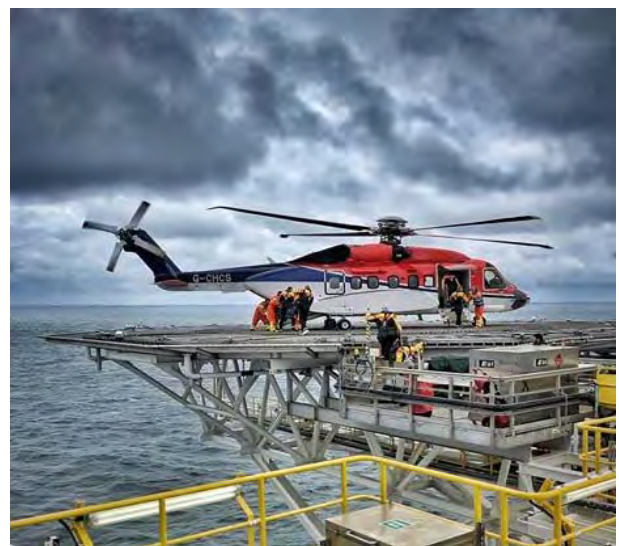
Figure 1: Offshore aluminium helideck
