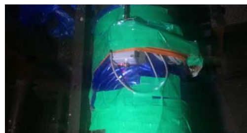
Figure 2: Telemetry system installation
