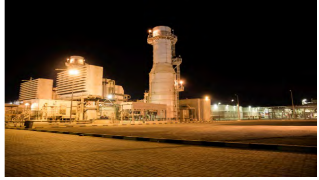
Figure 4: Frame 7 gas turbine power plant
