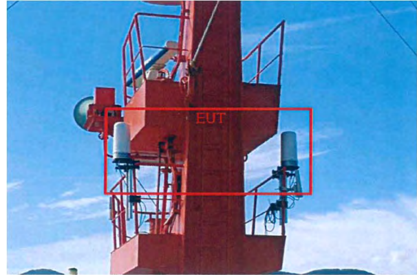
Figure 9: Sample installation of distance range test
