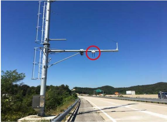
Figure 2: The road side station for WAVE communication
