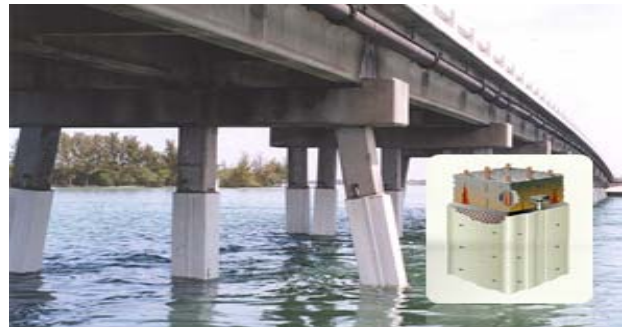
Figure 7: Zn-Mesh anode SACP system in FRP jacket
