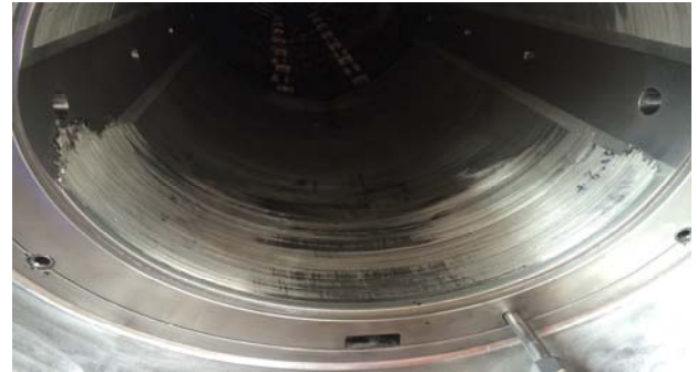
Figure 1: An example of damage of stern tube bearing due to misalignment
