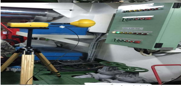
Figure 4: Measurement process of switch board
