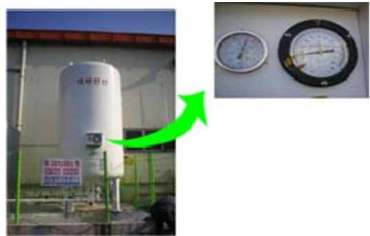
Figure 1: Analog Liquid gas level gauge
