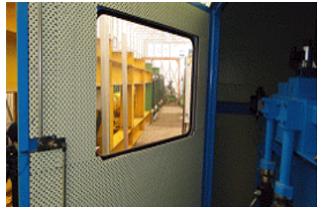
Figure 5: Internal feature of shield chamber covered by sound-absorbing materials
